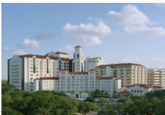
Memorial Hermann Hospital New Pavilion, Houston, TX
